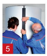
After attaching the cover strip, the thermal insulation can be closed by means of the second hook closure strip.
