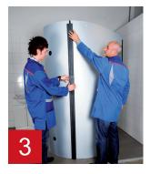
Lock the non-perforated thermal insulation part into place on the hook closure strip of the already attached thermal installation part.
