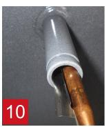
Installation of the sensor with accompanying immersion sleeve spring. A total of 3 sensors can be installed per immersion tube.
